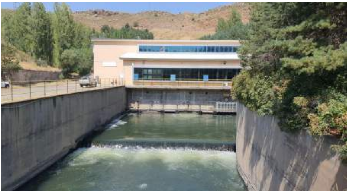
Photos 5 Facility building
