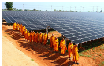
Nakhon Ratchasima Solar Farm Nakhon Ratchasima Province, Thailand
